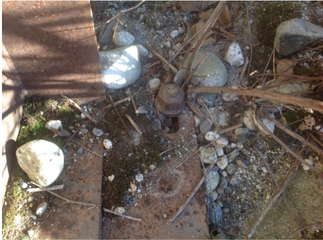
left bearing bolts at far end of slot
