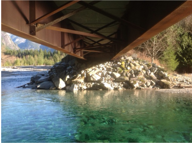
Left Bank Abutment when facing downstream
