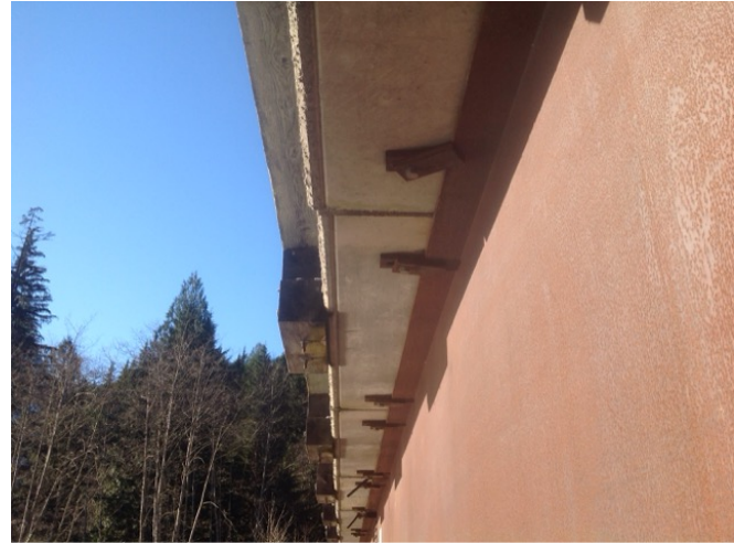
downstream deck clips
