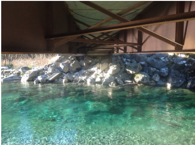
Right Bank Abutment when facing downstream
