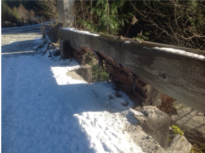
damaged guardrail
